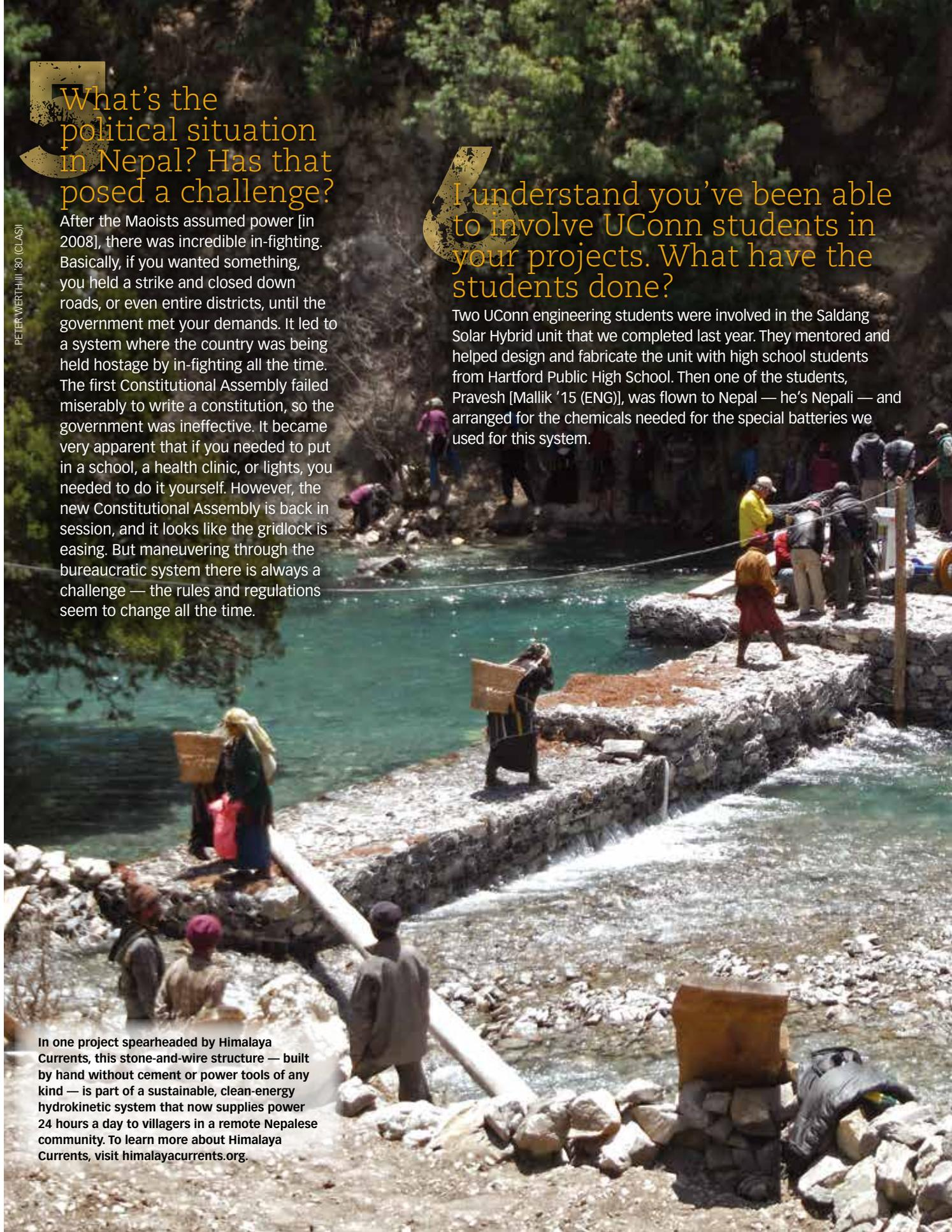
In one project spearheaded by Himalaya Currents, this stone-and-wire structure — built by hand without cement or power tools of any kind — is part of a sustainable, clean-energy hydrokinetic system that now supplies power 24 hours a day to villagers in a remote Nepalese community. To learn more about Himalaya Currents, visit [himalayacurrents.org](http://himalayacurrents.org).
